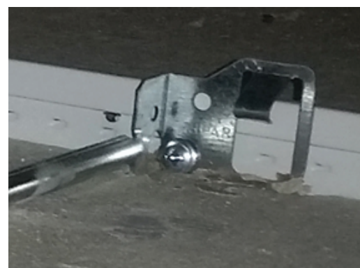
Figure 4: Screw mounting example
