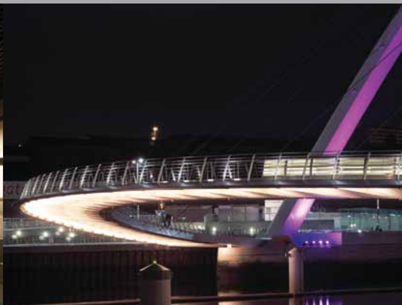
Millennium Bridge, Gateshead, Inglaterra
