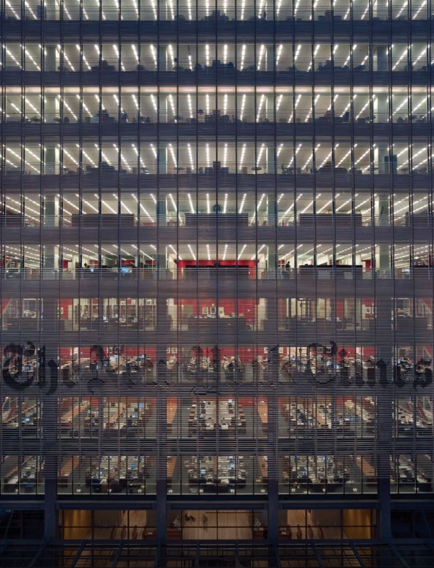
The New York Times Building uses Quantum® to increase comfort and productivity while saving energy ( www.lutron.com/nyt ).
