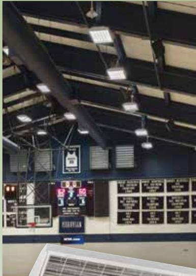
Lutron High Bay Athlite™ fixtures were used to replace existing HID fixtures, reducing the connected load by 48 percent.
