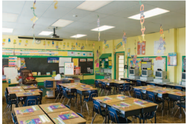
Balance LC dims rows of lights to different levels to take advantage of natural light while providing even illumination on student desks.
