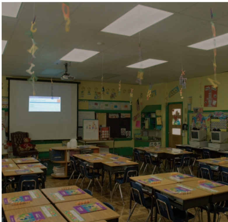
After: Balance LC from Lutron provides dimmable control of the fixtures, reducing glare, making presentations easy to see.
