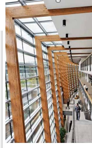
■ LEFT: The south-facing atrium at SAP Americas includes a brise soleil to reduce sunlight entry. RIGHT: Since lighting is by far the largest user of electricity in commercial buildings, including a combination of lighting controls and daylighting in a workspace limits energy consumption.
