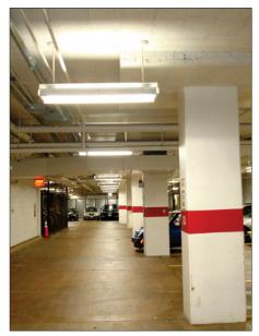
By replacing this legacy lighting system with new fixtures, dimming ballasts and occupancy sensors, one State Department building garage saved more than 400,000-KWh, or about \$64,000 in electricity costs, annually—an estimated 83 percent energy savings from the baseline.
