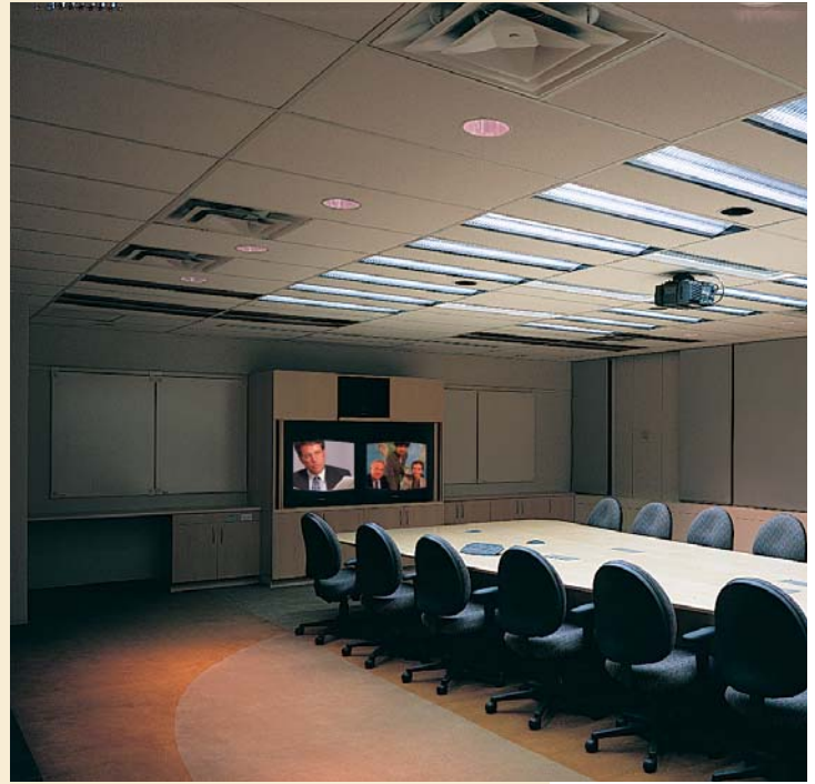
Scene 2: Teleconferencing – the lighting is relatively high, with proper balance of brightness on the ceiling, side and end walls for video camera. Participants' faces and upper bodies are illuminated by ceiling fixtures that are angled for asymmetric distribution of light. Window shades are blacked out.
