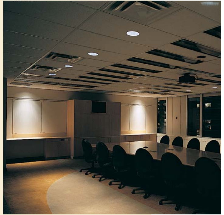
Scene 4: Unoccupied/Nightlight – Accent lighting washes the back wall and walk area of the room. Window shades can be up or down.
